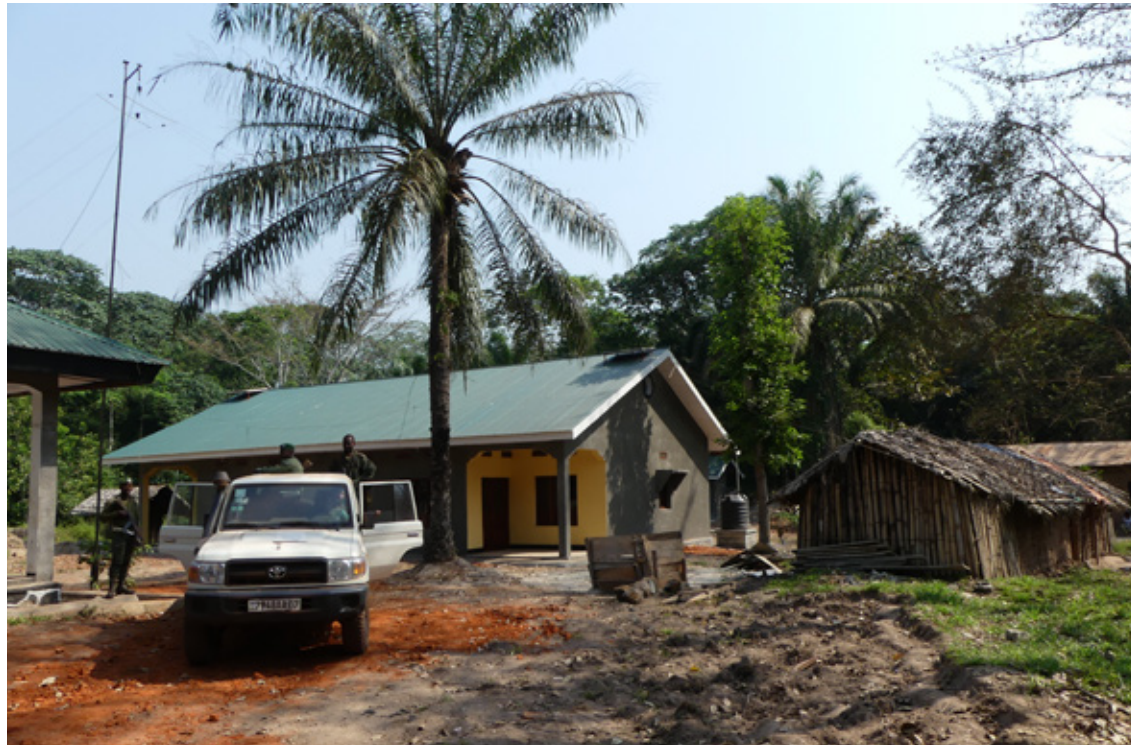
Newly built ranger accommodation block at Adusa outpost in Okapi Game Reserve in the Democratic Republic of Congo, funded by the ECF. The old accommodation is on the right of the photo. © Chris Thouless.
