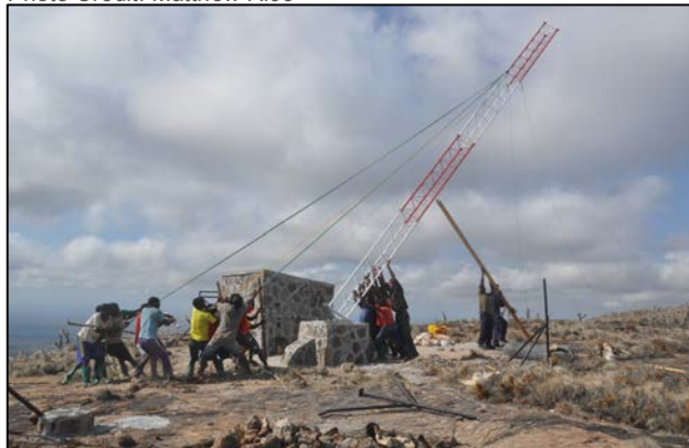
Digital radio network being installed in Niassa National Reserve, Mozambique.
